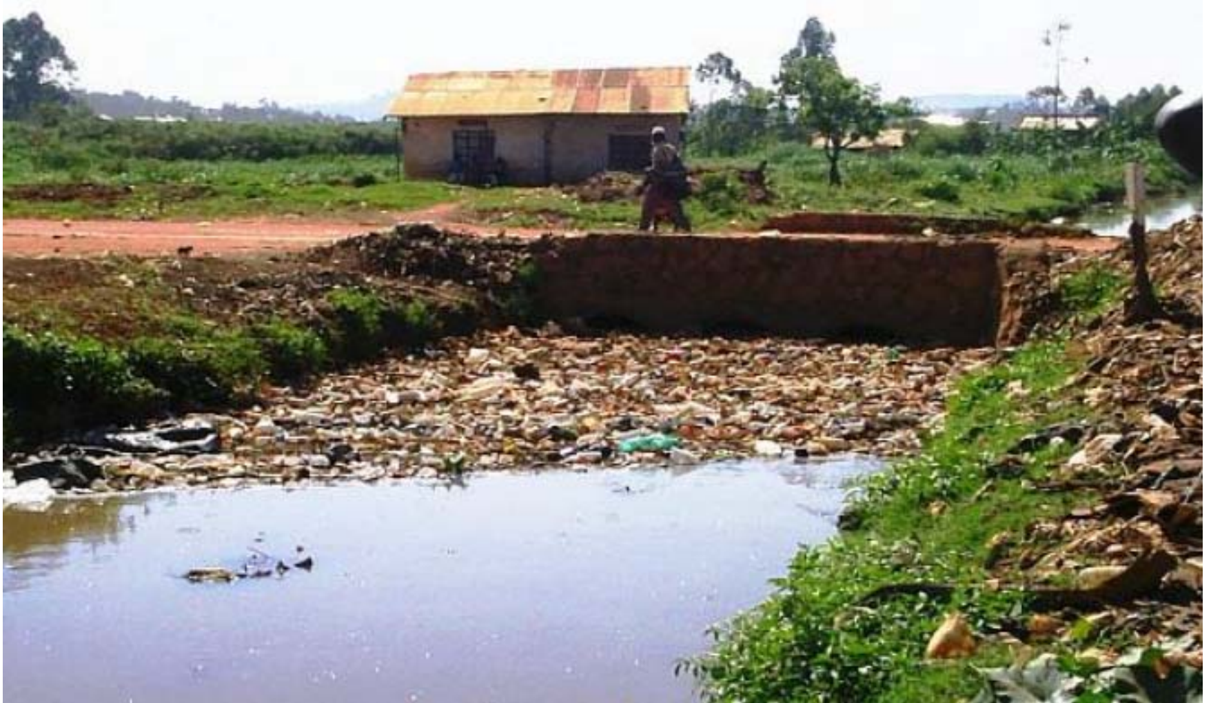
Solid wastes piling at culverts along Kawala road crossing of drainage investments
