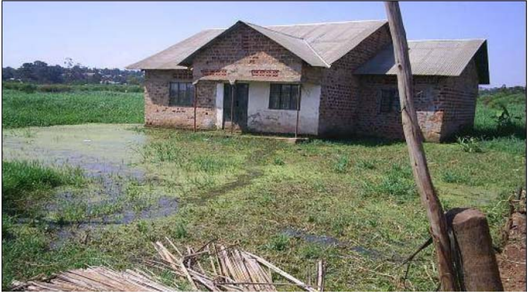
House in Lubigi swamp, Bwaise, next to Nsooba Channel
